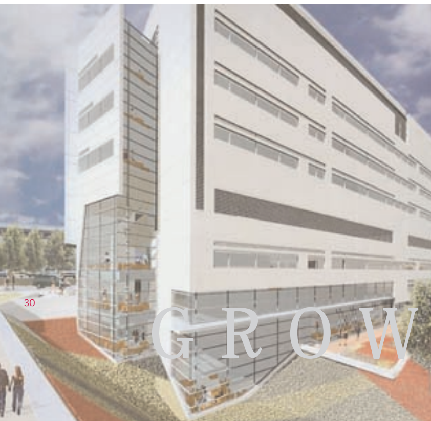
New Jersey Medical School-University Hospital Cancer Center
