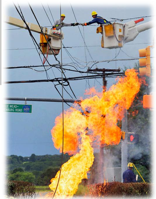
PSE&G crews in NJ work on restoring power as flames from a ruptured gas main shoot high into the air. A bolt of lightning from a strong thunderstorm hit the utility pole bringing down a power line. The electricity arced to the gas pipe and ignited it.
